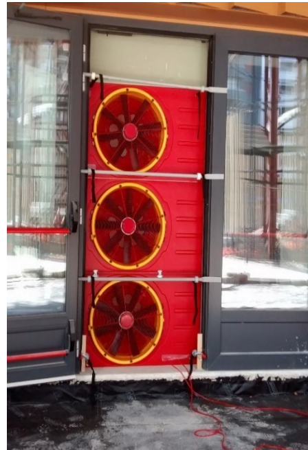
Figura 9. Test de Blower Door.
