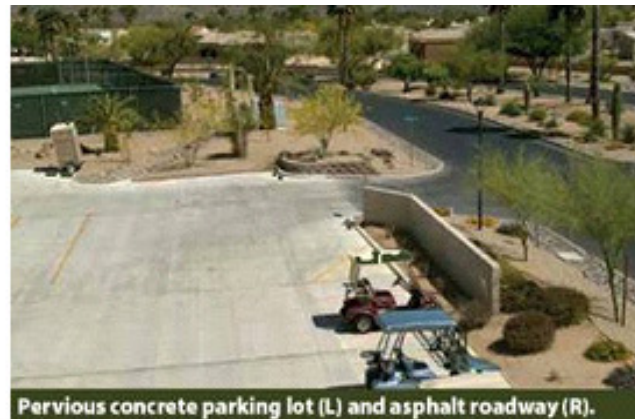
Pervious concrete parking lot (L) and asphalt roadway (R).
