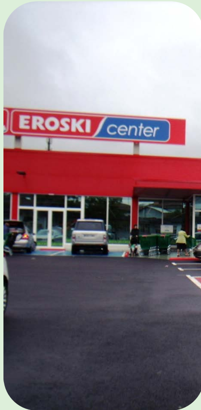
Supermercado Eroski Center, Oñati
