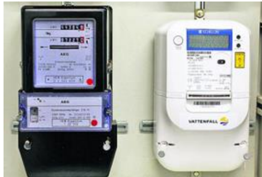
Figure 21 Electric energy meters.
