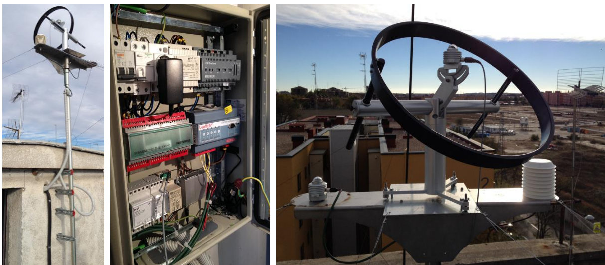
Figure 52 – Weather station installed
