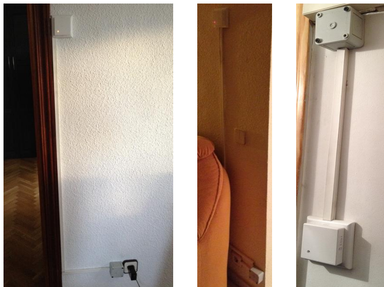
Figure 51 – Comfort sensors installed in B2/F4/D1
