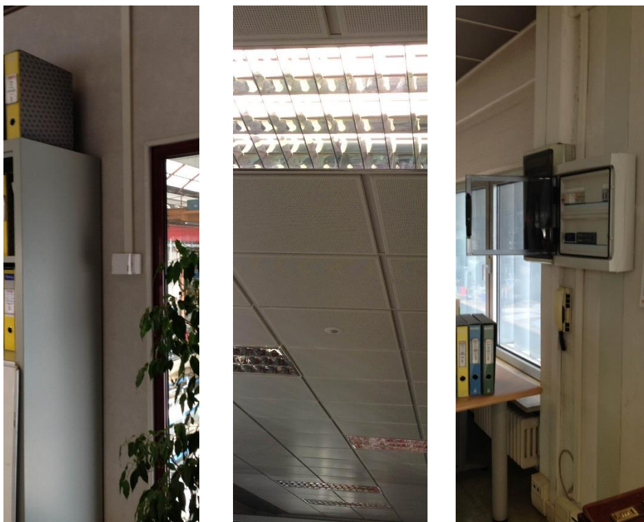
Figure 58 - Comfort sensor (left), brightness sensor (center) and receiving station (right)
