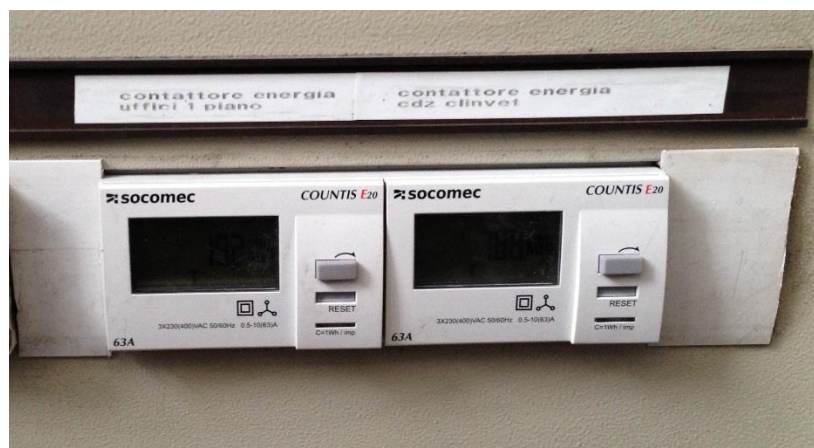
Figure 57 – Electric meters installed
