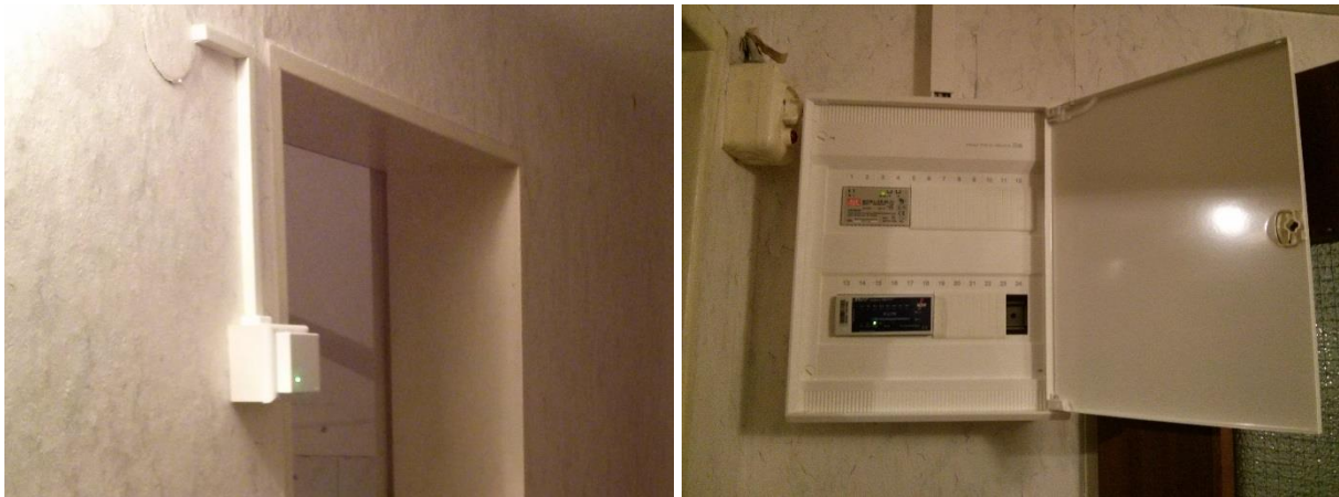
Figure 56 – Comfort sensor (left) and receiving station (right) in the cellar floor
