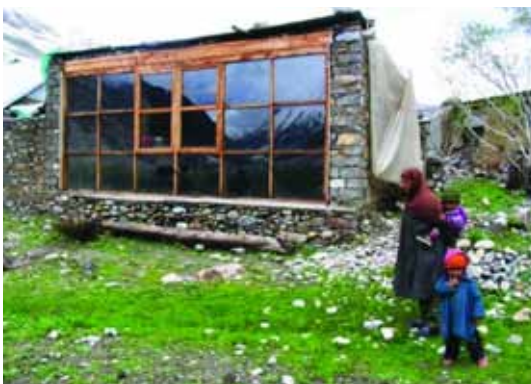
Solar wall in Kargil District.
