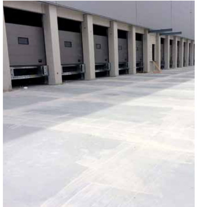
MasterFiber 246 Pavimento industrial, Madrid
