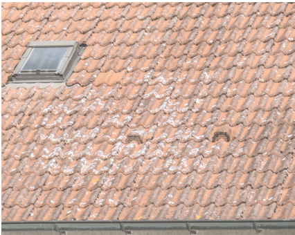
Damp through penetration/roof
