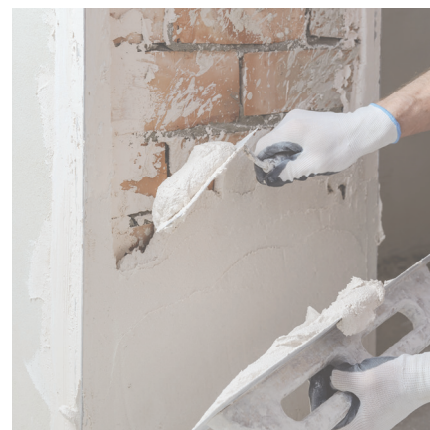
Re-coating with breathable plaster
