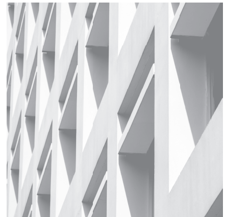
Waterproofing concrete and cement façades
