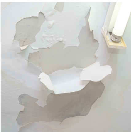
Damp through penetration/leak
