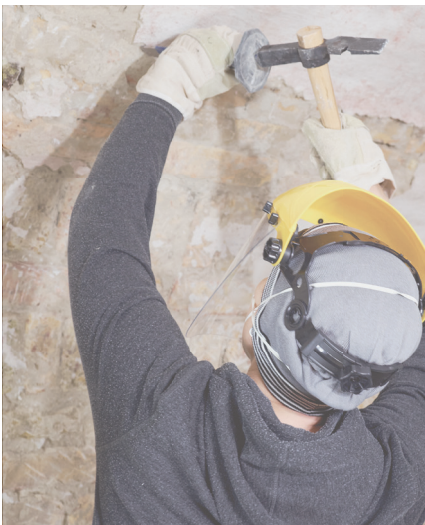
Chipping/removing layers or coating
