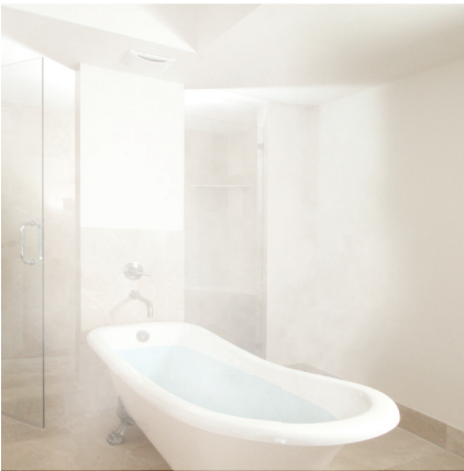
Condensation damp. Steam
