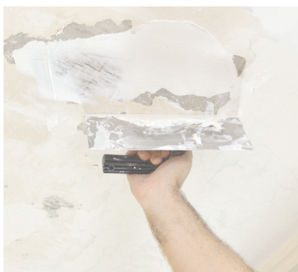
Crack Filling
