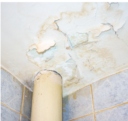
Damp through penetration/ rupture
