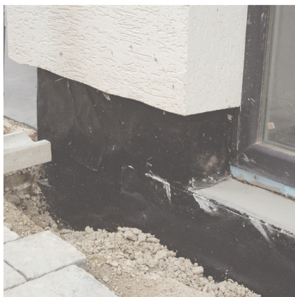
Exterior waterproofing with Brea (Pitch)
