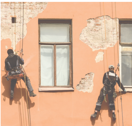
Damp through penetration/ façade
