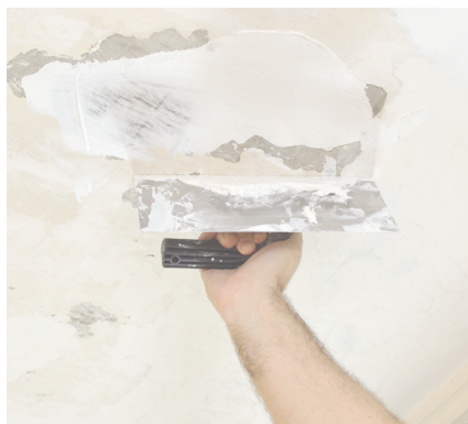
Crack Filling
