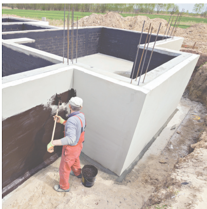
Exterior waterproofing with Brea (Pitch)
