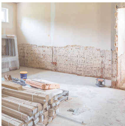
Wall exposed for evaporation
